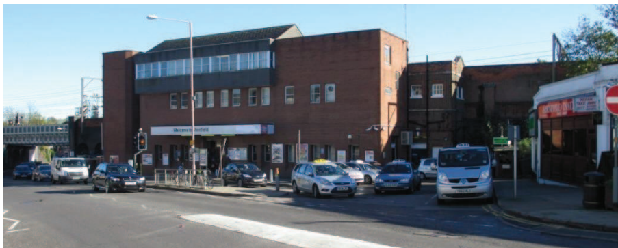
Figure 2-5: Shenfield Station Forecourt Area from southwest perspective
